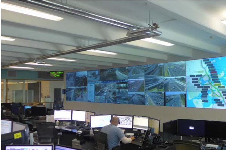
Figure 2-34: Auckland Traffic Operations Center control room.
