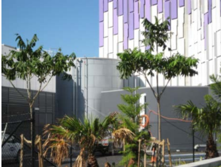
Figure 2-6: Clem7 (Brisbane, Australia) Tunnel water storage tank.
