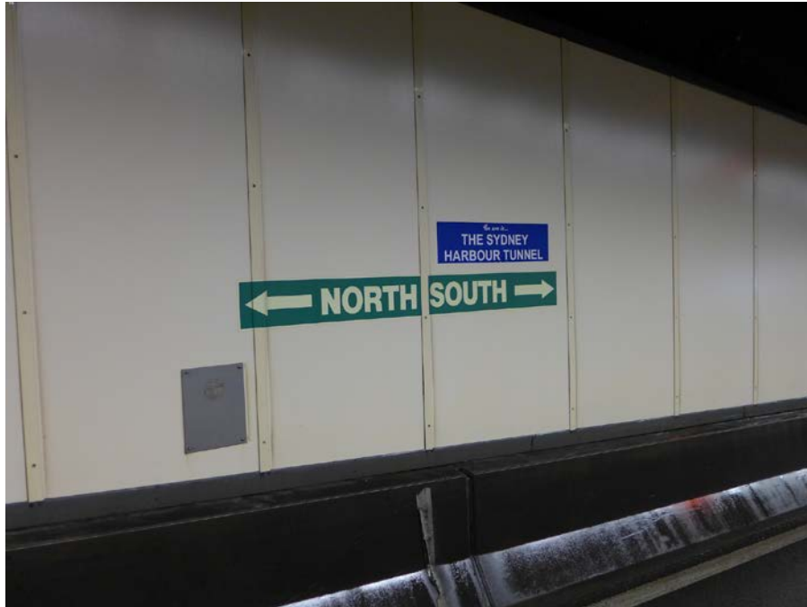
Figure 2-19: Sydney Harbor Tunnel location signage.
