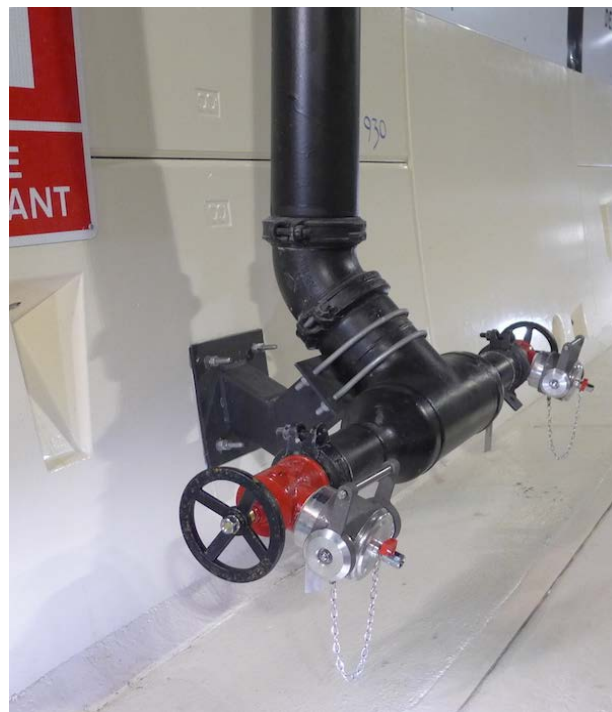
Figure 2-32: Waterview Tunnel fire hose attachment detail.
