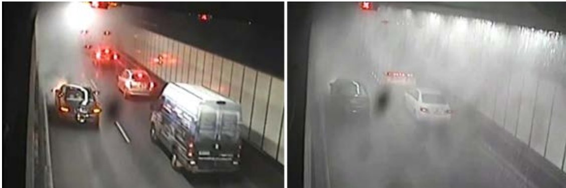
Figure 2-44: M5 East car fire inside of tunnel, prior to FFFS activation (left) and during activation (right).
