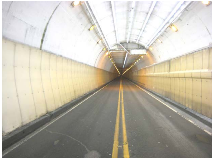
Figure 2-24: Mount Victoria Tunnel prior to rehabilitation.
