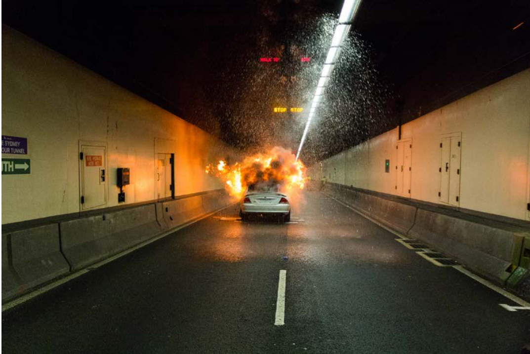
Figure 2-47: Sydney Harbor Tunnel live fire and FFFS demo at start of FFFS activation.
