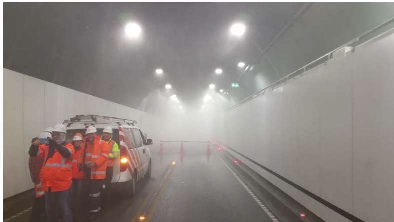
Figure 2-7: Water droplet drift due to wind in the Mount Victoria Tunnel (upstream boundary of FFFS zone at traffic cones).
