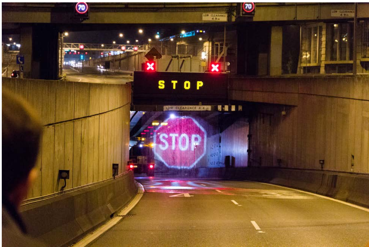
Figure 2-55: Sydney Harbor Tunnel water stop sign projection.
