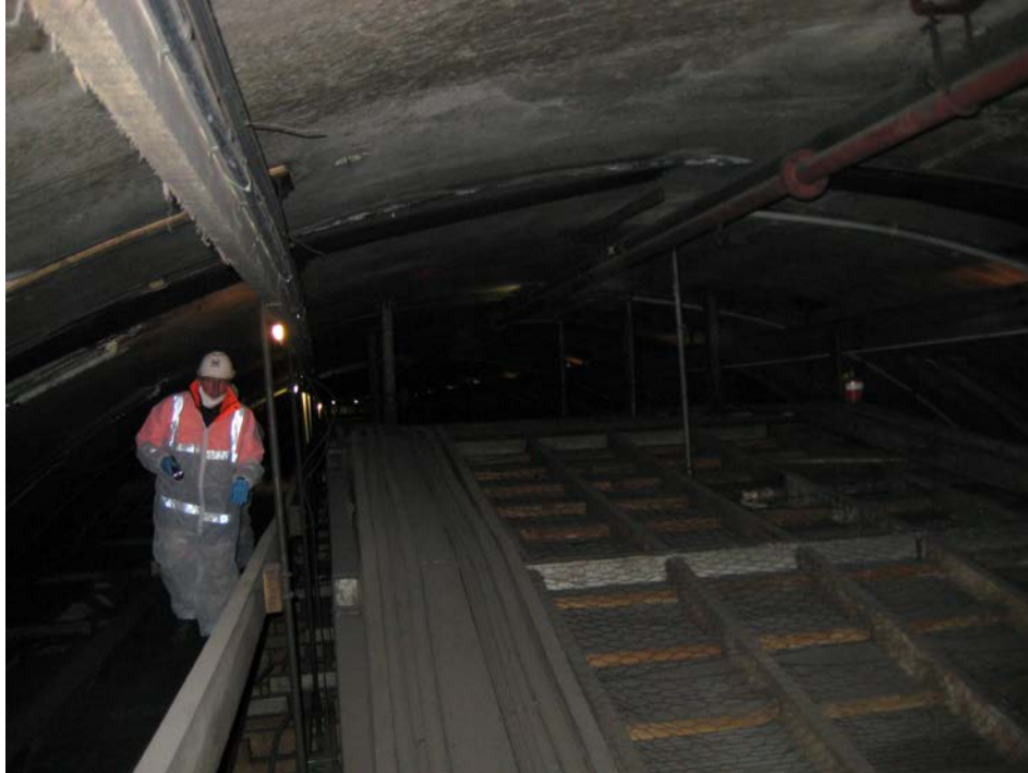
Figure 2-21: Terrace Tunnel wooden ceiling plenum prior to rehabilitation.
