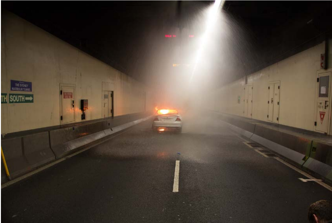
Figure 2-49: Sydney Harbor Tunnel live fire and FFFS demo about 1 minute after FFFS activation
