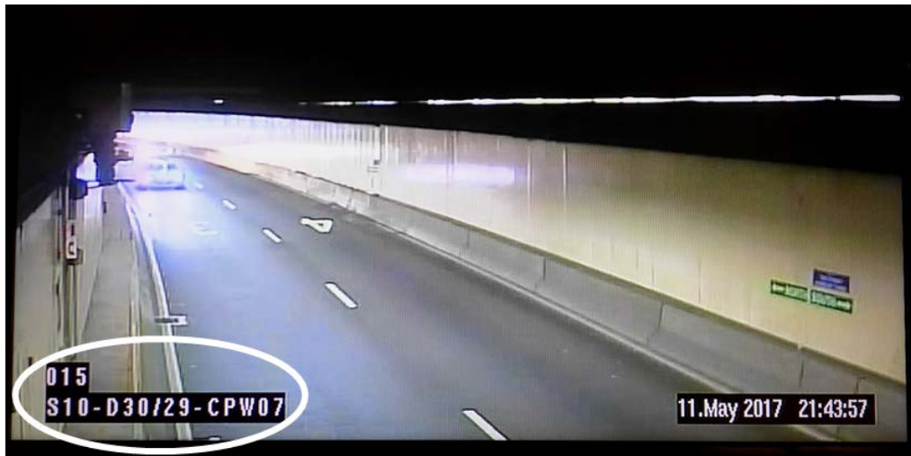
SOUTHBOUND TUNNEL DELUGE ZONES 30/29 CROSS PASSAGE 7
