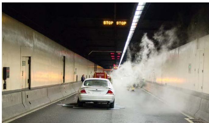
Figure 2-38: Sydney Harbor Tunnel fire test showing traffic control signage.
