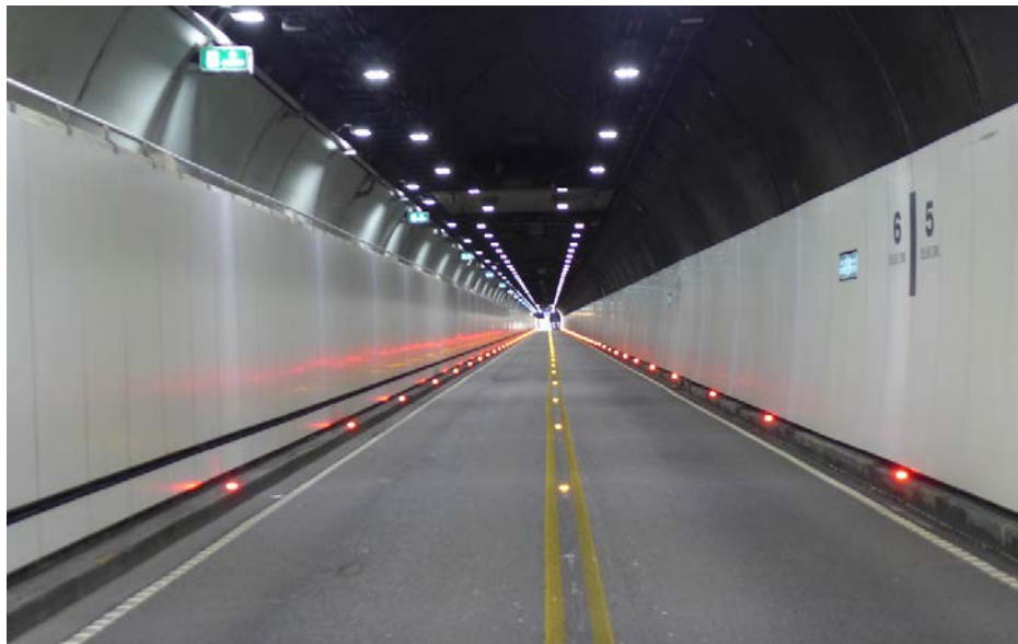
Figure 2-65: Mount Victoria Tunnel roadway marking lighting demonstration.
