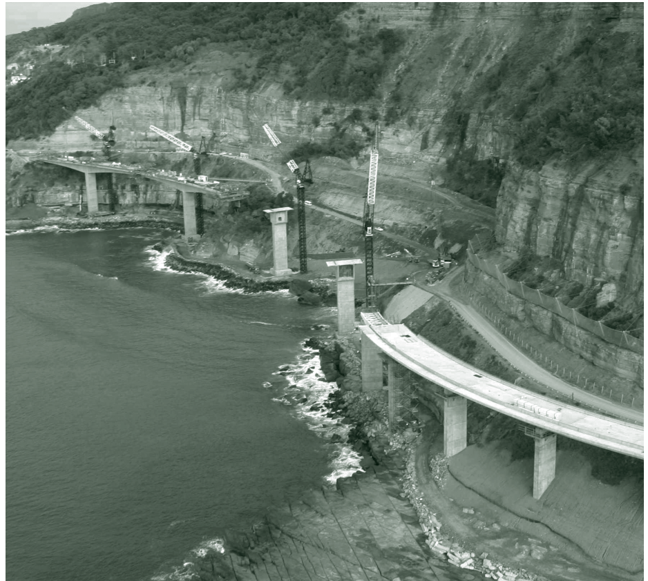
Figure 6. Seacliff Bridge project in New South Wales.
