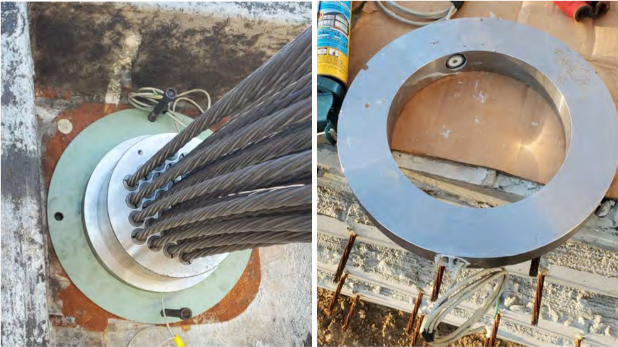
Figure 9: Field implementation of the VCensors. (Source: VSL International)
