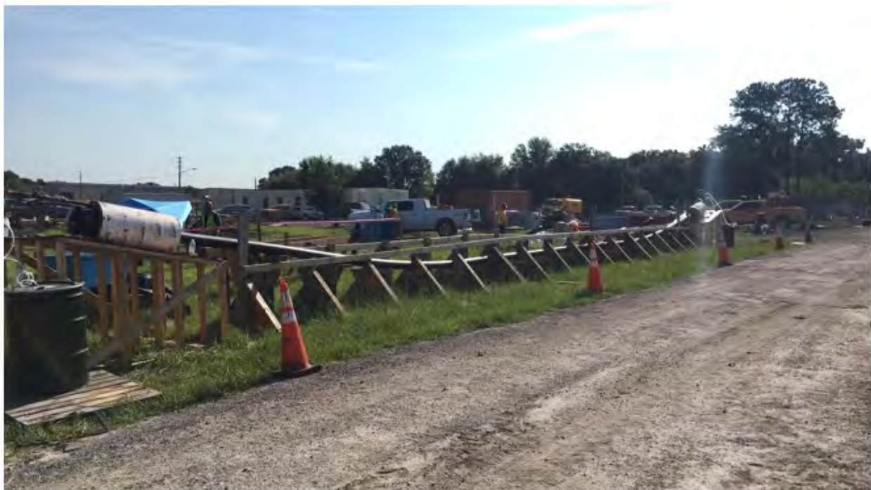
Figure 17: Pre-construction tendon mock-up (Source: FDOT)
