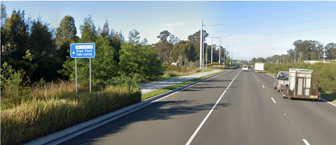
Figure 38: Northern Road, Oran Park, New South Wales Source: Google Street View (84)
