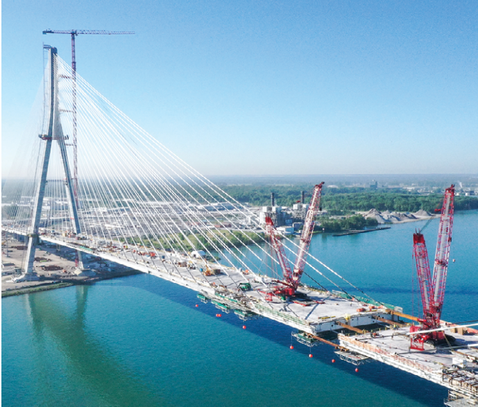
Final preparations for the bridge deck closure (Photo: Detroit Bridge Authority)
