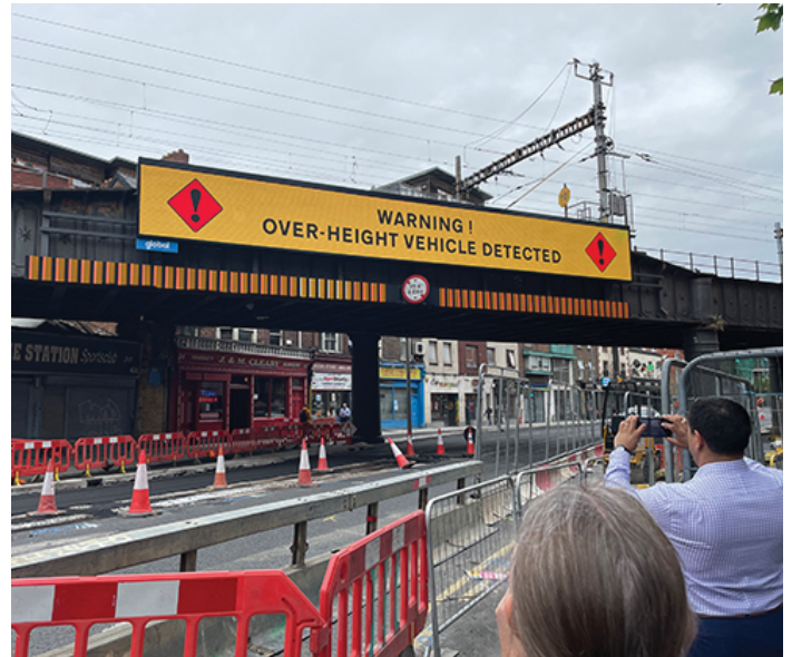
View of Irish Rail warning system triggered by an over-height vehicle (Photo: FHWA)
