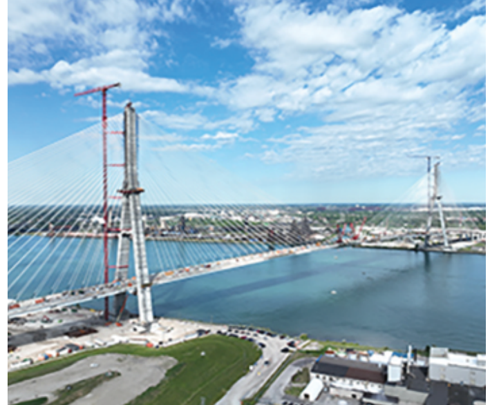
Completed deck closure view from Canada into the US Windsor (Photo: Windsor Detroit Bridge Authority)
