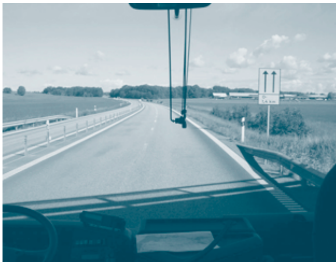
Figure 7. 2+1 roadway. Note the cable barrier and sign indicating the length of the passing lane. (Sweden)
