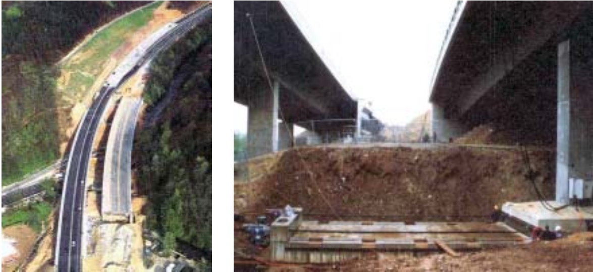
Figure 11. Jacking a bridge into final position (from German presentation).
