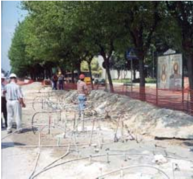
Figure 16. Turin subway grouting project site visit showing: (a) grouting and (b) grout pump station.
