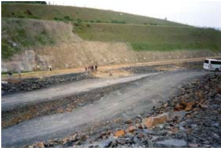
Figure 8. Field visit to Meschede roadway slope stabilization project.
