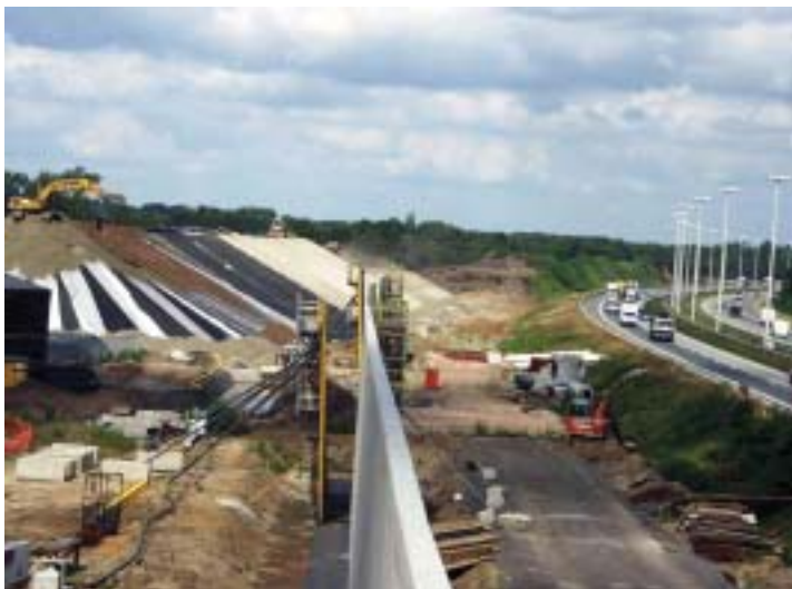
Figure 19. Sound barrier construction using capped debris and contaminated soil mound.
