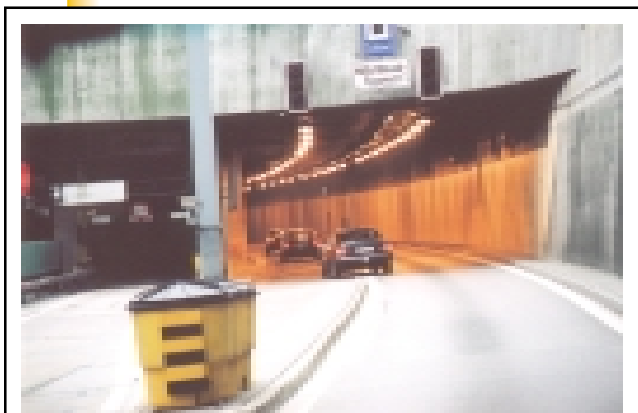
Figure 29. Milchbuck Tunnel, Switzerland.
